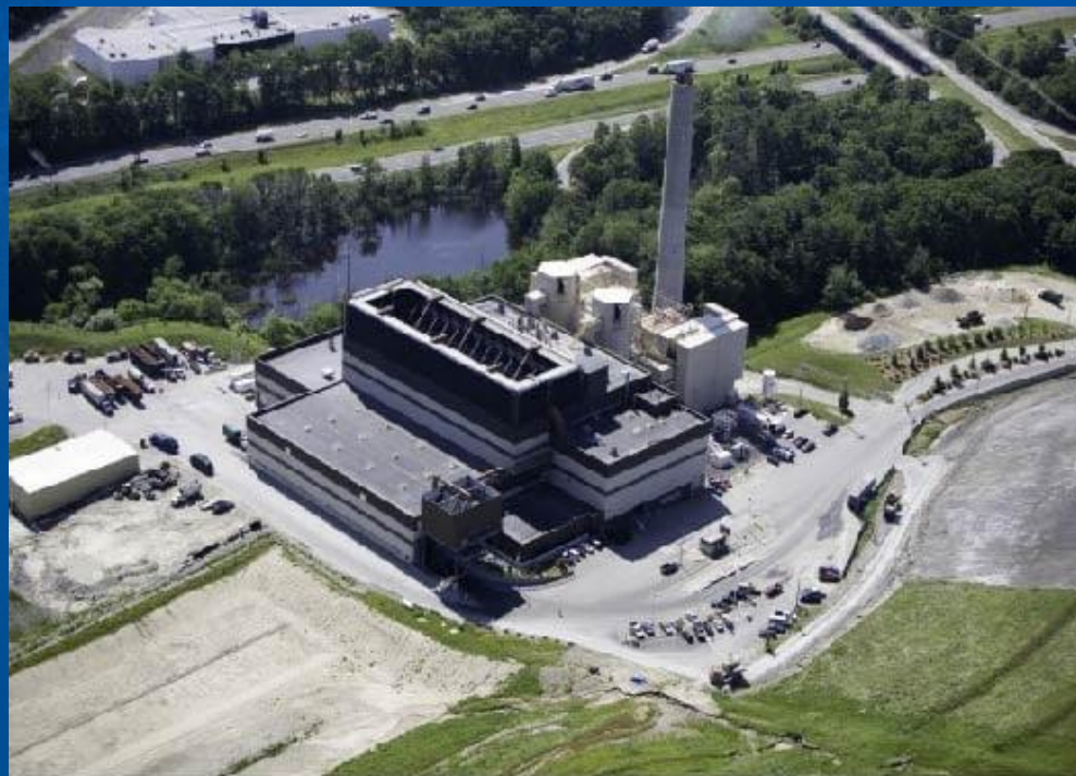
Haverhill WTE Facility – 1,600 TPD
